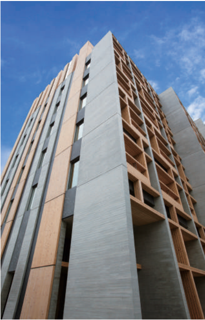
The concrete and steel structural framework is covered with Japanese cypress lumber that creates a consoling and friendly appearance.
