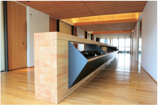
The space between the small hall and the meeting rooms has a showcase for displaying a “Collection of Wooden Crafts from Around the World.” The showcase is made from Japanese cypress boards that have been layered together.
